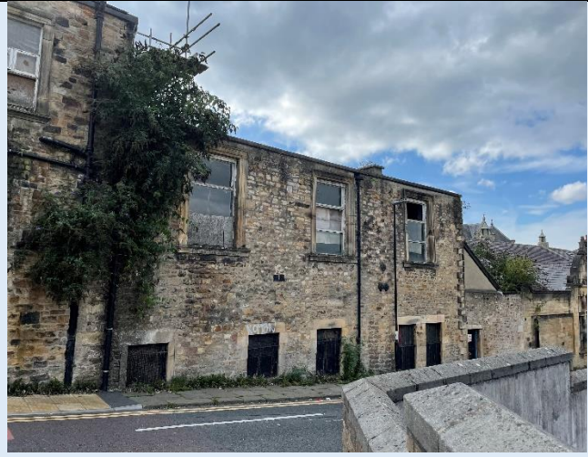
Figure 8: East elevation, Phoenix Street (former first floor chapel alterations, north elevation (C. Stansfield) now has a flat roof, and the arched windows altered)
