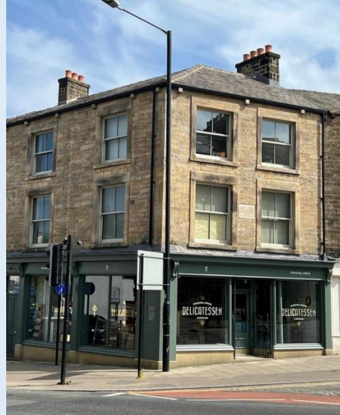
Figure 13: Following the completion of phases 1 & 2 (May 2023)
