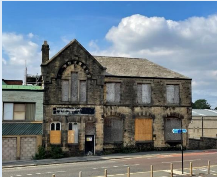
Figure 1: 50 St Leonard's Gate, on the corner of Phoenix Street
