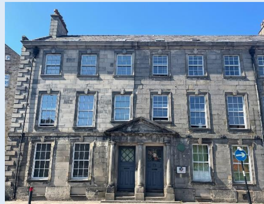
Figure 5: 1-3 Cable Street, Lancaster
